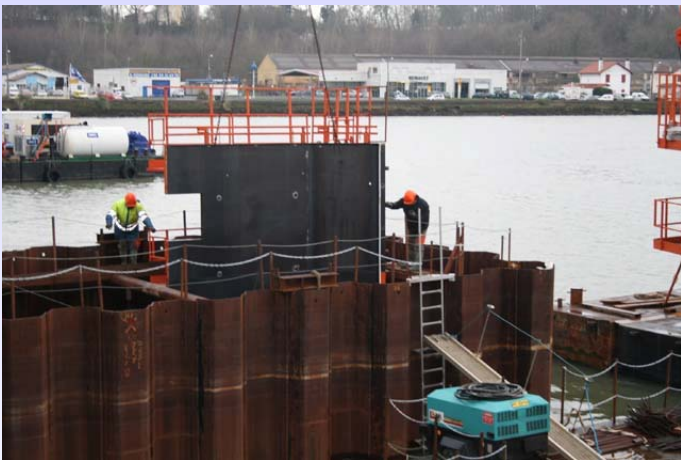
Position of the scaffolding to P7 stack elevation
